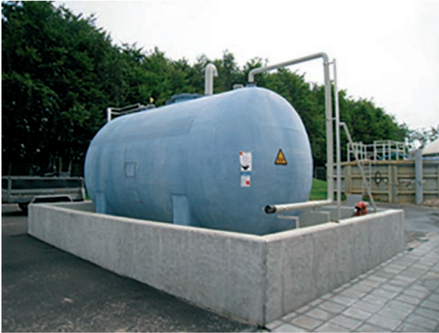
FIGURE 5.6 Storage tank installation for iron chloride. PHOTO Kemira.
